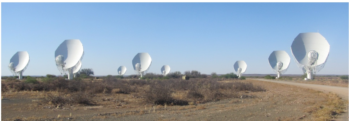
Figure 3.2. View of nine of the 64 antennas that compose the MeerKAT radio telescope array. Photo credit: Alessandro Ridolfi (2018).
